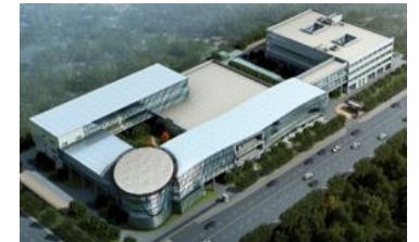
R&D center, Shanghai Anting
