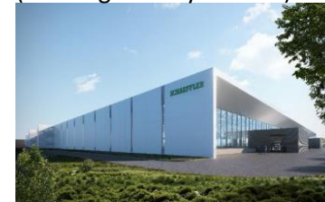
Xiangtan – new campus (Building 1 ready in 2019)
