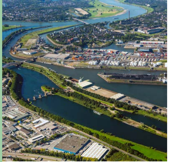
The Duisburg Inner Harbor depicted here is the largest of its kind in the world. It’s the hub for the Rhine and Ruhr rivers and several artificial waterways
