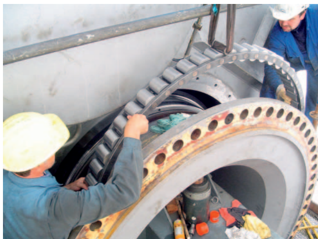
FAG and Tenova TAKRAF fitters mounting one of the cage segments
