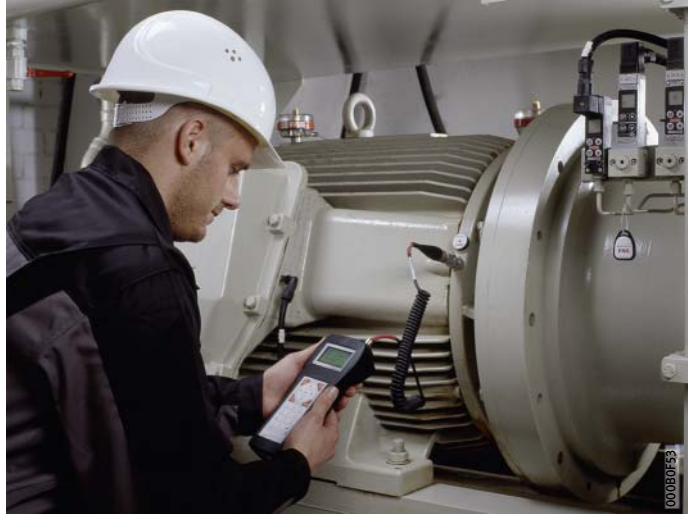
Figure 14 Independent checking of machine condition
