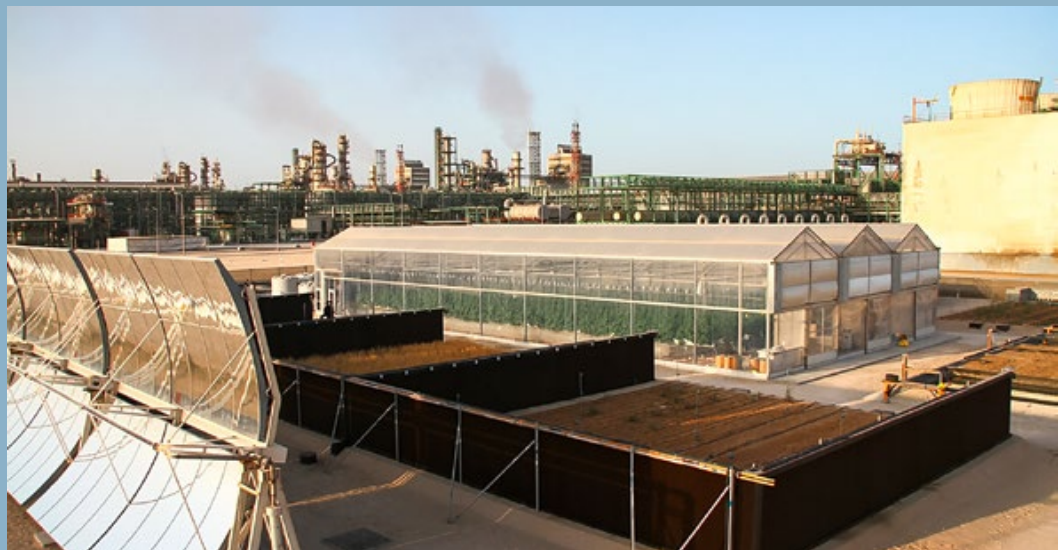
Cooling greenhouses that produce freshwater
