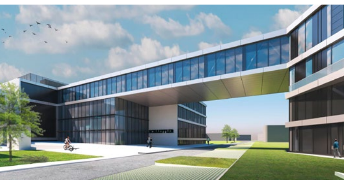
Investment in transformation: A new competence center for electrified mobility is being established at the headquarters of the Automotive Technologies division in Bühl
