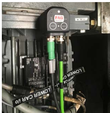
Schaeffler’s SmartCheck online measuring system monitors the sorting machines at Royal Mail
