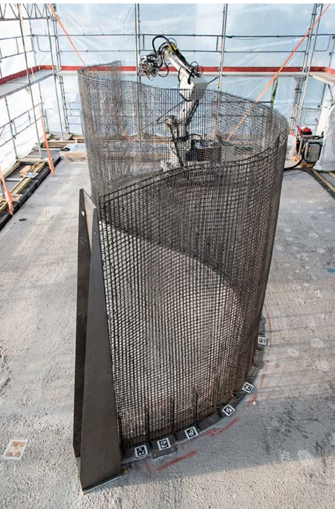
An industrial robot (in situ fabricator) fabricates a 3D grid structure filled with a type of concrete that has specific flow characteristics
