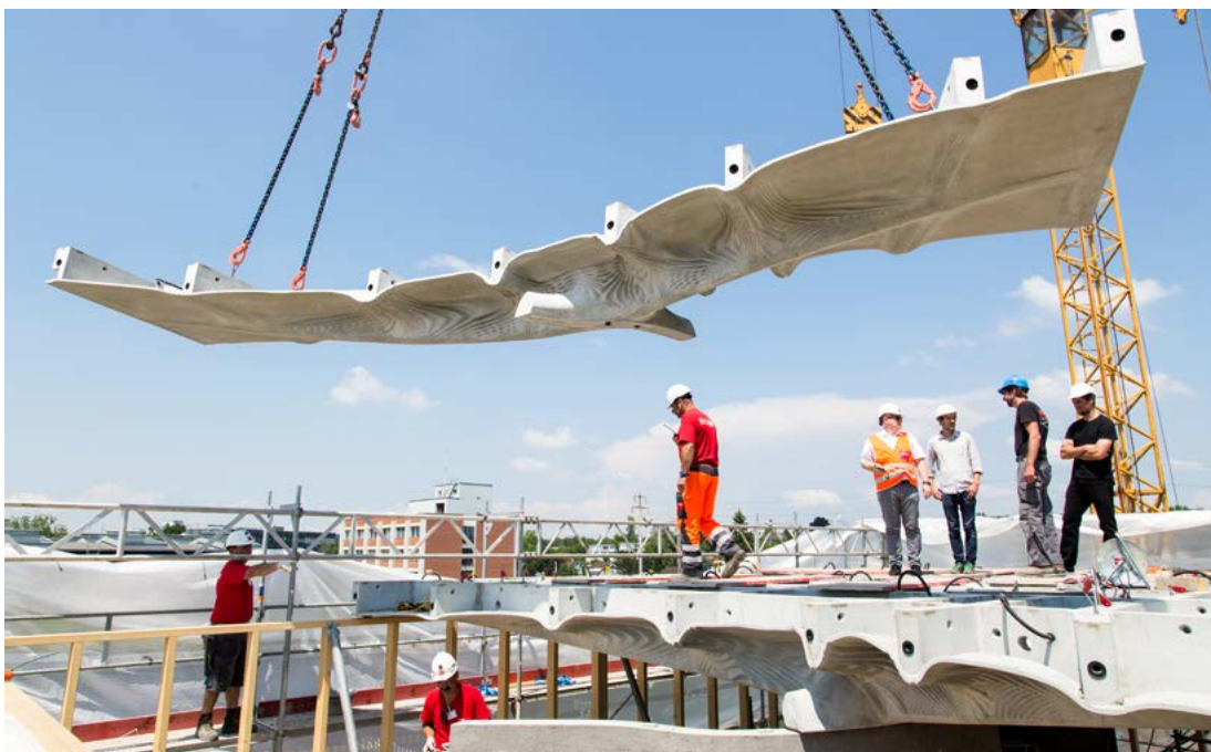
Digitally planned, additively manufactured: The curved ceiling elements that were cast in a 3D-printed casing are joined together at the construction site
