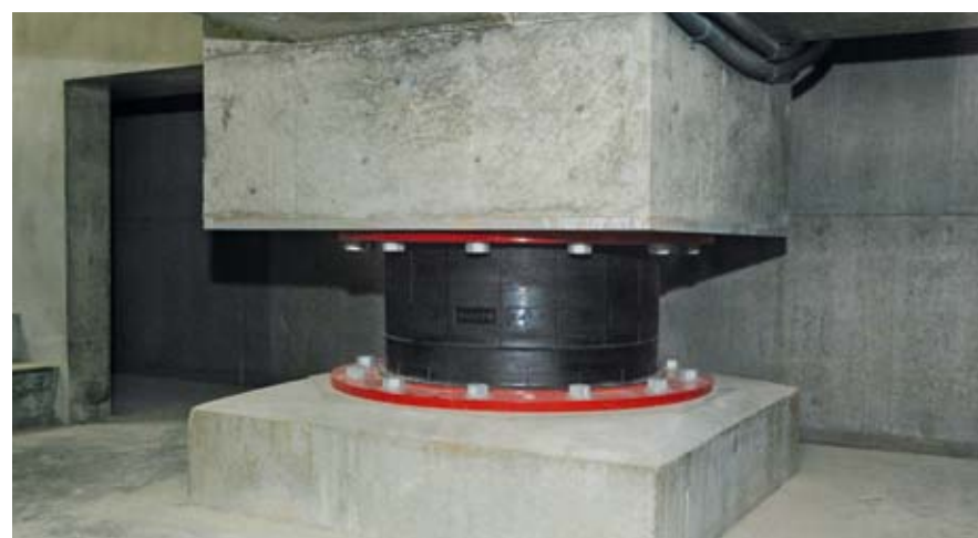
Earthquake-proof structure: Damping elements in the building's foundations
