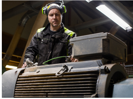
Commissioning of the SmartCheck on the main motor
