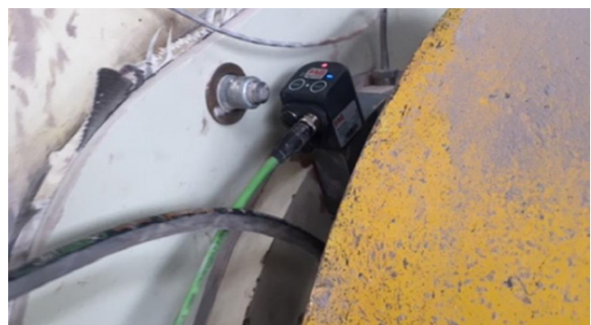
SmartCheck installed on the bearing housing
