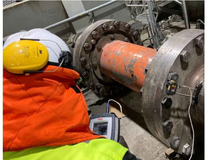
Alignment of the shaft with the alignment system LASER-EQUILIGN in the old design. Successor is the LASER-EQUILIGN2 with improved design, more functions and even more precise technology.
