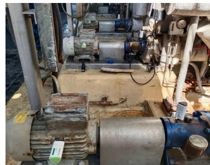
OPTIME sensors on pumps
