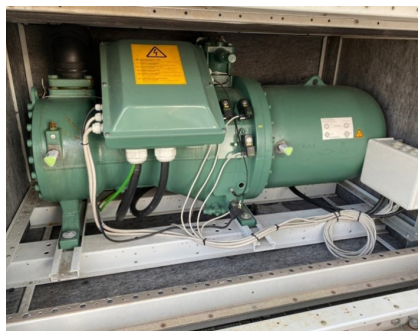
OPTIME sensors on a chiller compressor
