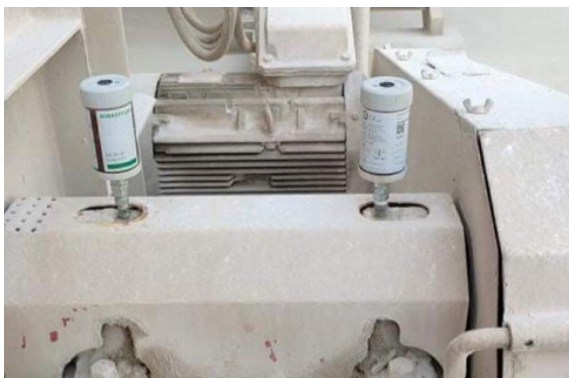
CONCEPT1 – Machines are lubricated with the right quantity of grease at the right time.
