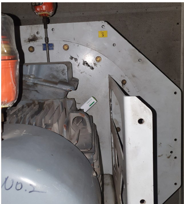
The OPTIME sensor on the motor of a cooling fan detected the changed machine status.
