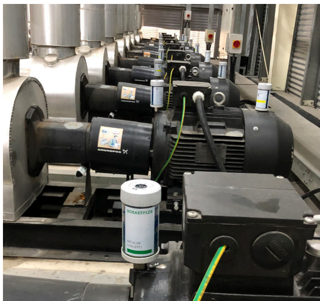
CONCEPT1 are installed on motors and pumps.
