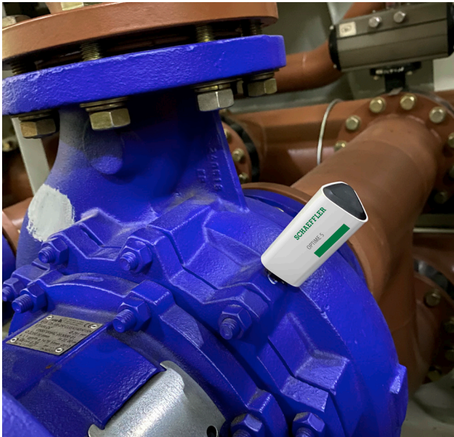
Schaeffler OPTIME sensor on a motor
