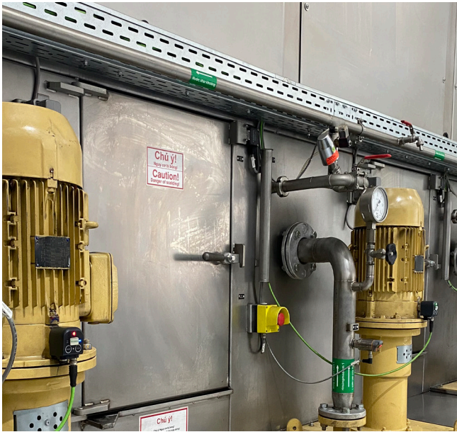
SmartChecks installed on critical pumps.
