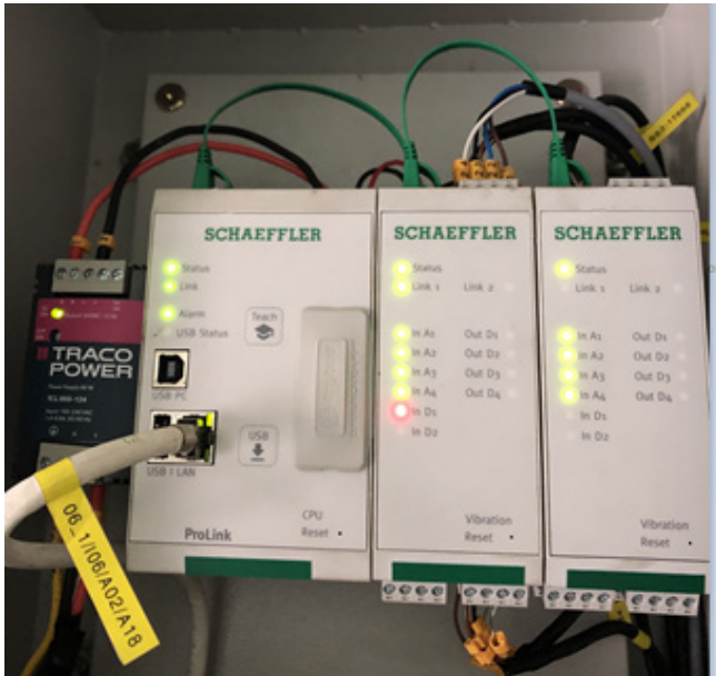
Schaeffler ProLink CMS in the control cabinet
