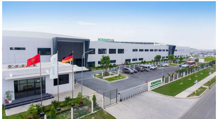
Schaeffler plant in Bien Hoa City , Vietnam
