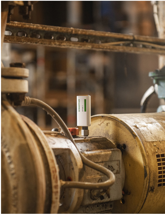
OPTIME sensor on a pump
