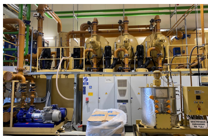
Central oil supply system
