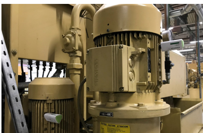
OPTIME on motors of an emulsion pump
