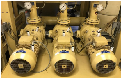
OPTIME sensors on KSB motors
