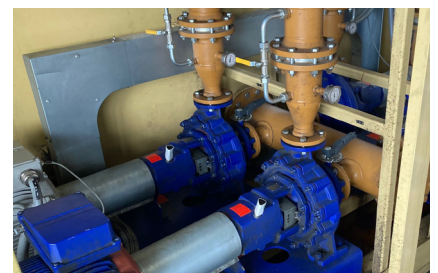
OPTIME on main oil supply system pumps
