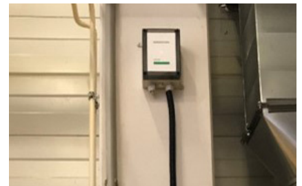
Gateway installed on the wall
