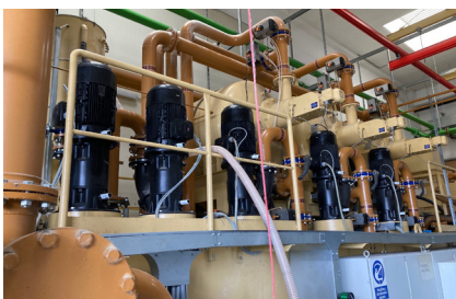
OPTIME on oil supply system pumps
