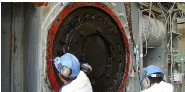
Maintenance work on the HPGR
