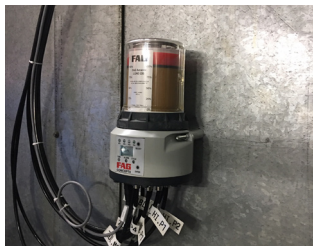
CONCEPT8 ensures precise lubrication of the bearings.
