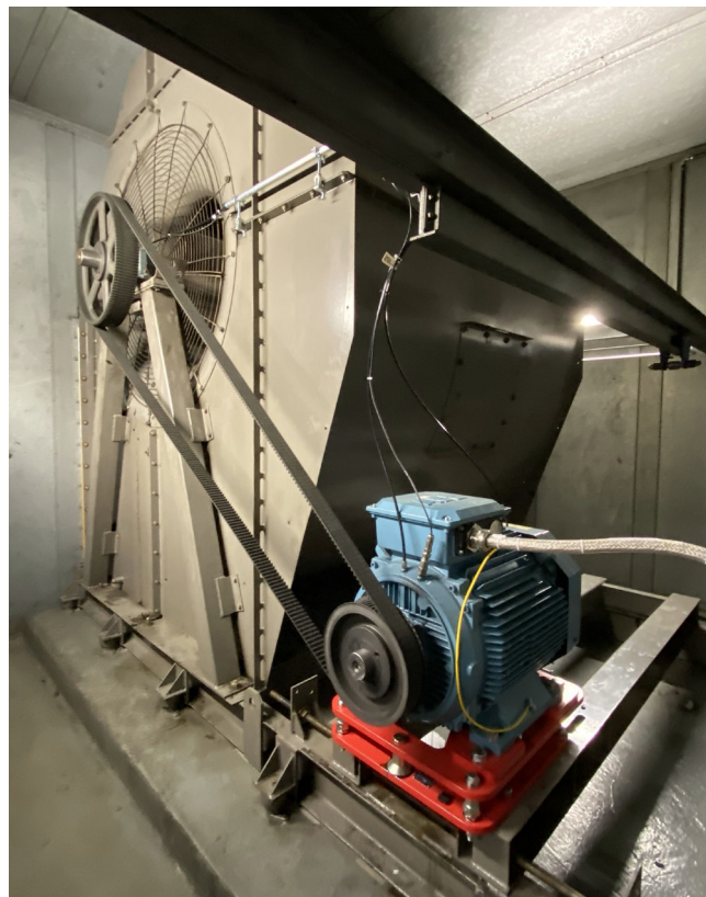
Fan with patented 3D motor slide and toothed belt drive at the automobile manufacturer's plant
