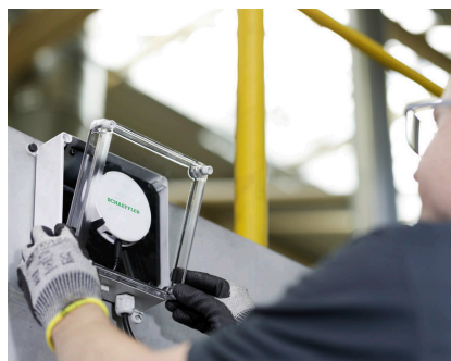
The gateway is mounted on the wall.
