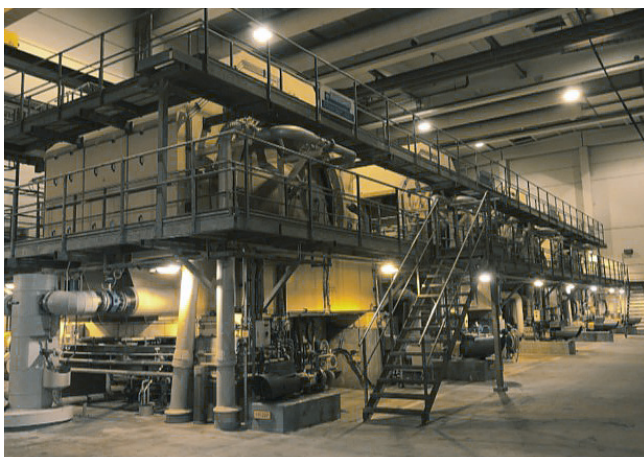
Sunila Mill , interior view
