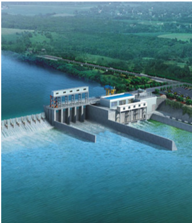
The dam regulates the water level of the region.
