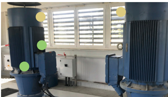
Motor monitoring with SmartCheck and lubrication system CONCEPT2
