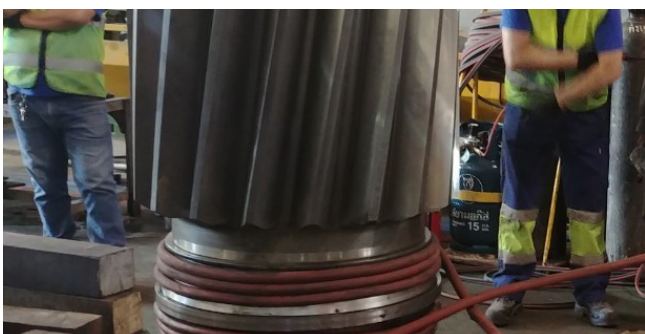
Bearing dismantling by heating leftover bearing inner ring on the shaft
