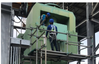
Workers preparing the SmartCheck installation.
