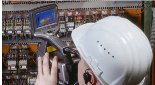
Switchgear is examined with a thermal imaging camera
