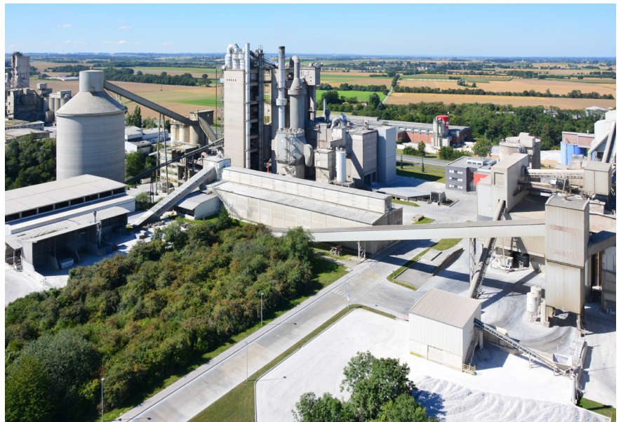
The Spenner site in Erwitte produces cement, lime, and dry mortar
