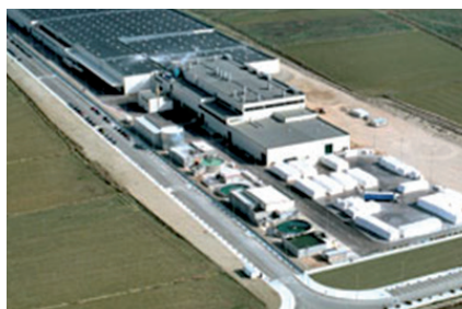
Plant in Spain
