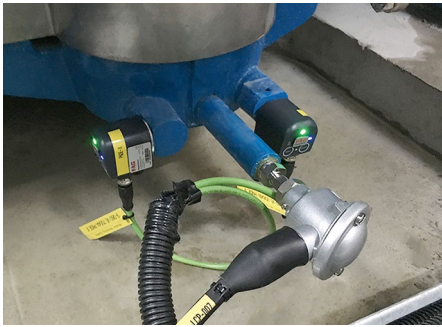
SmartChecks monitor all the important units in the pump stations
