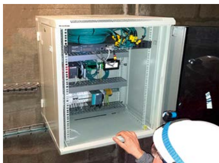
Control cabinet with SmartController
