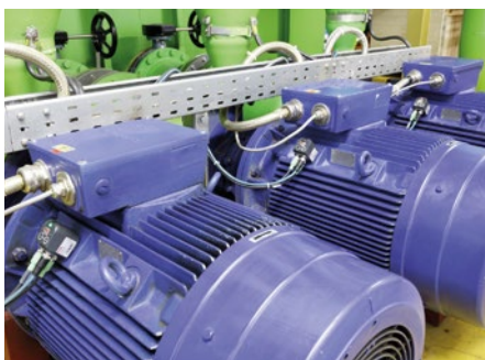
Monitoring of electric motor by FAG SmartCheck
