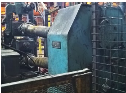
Monitored specialized gearbox
