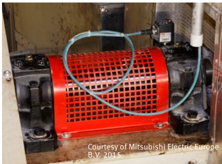
Ventilation unit: The FAG SmartCheck is fitted to the shaft's bearing support
