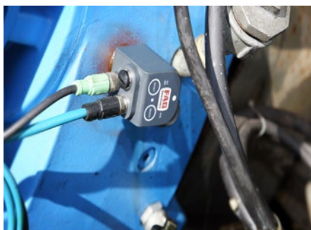
FAG SmartCheck measures gear vibrations
