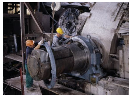
Fitters working on-site
