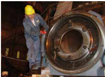
Mounting work at bearing housing
