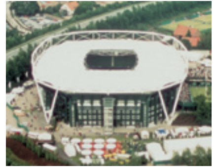
Stable but with flexible joints: roof design of the Gerry Weber Stadium in Halle (Westphalia, Germany)
