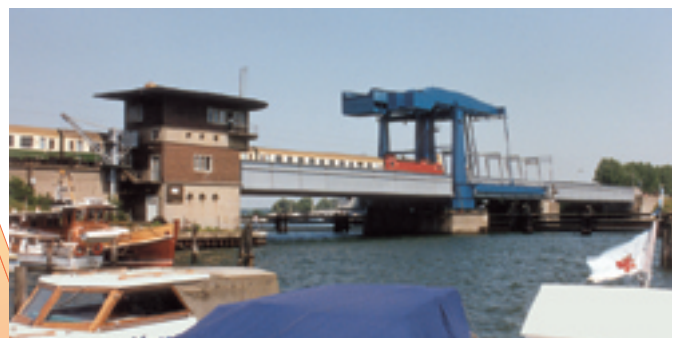
The Rügen causeway in Stralsund, Germany: The bascule bridge section is equipped with ELGES spherical plain bearings
