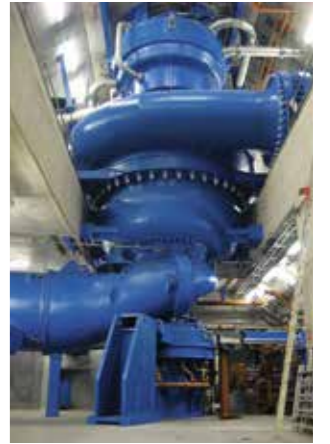
Pumped-storage power plant
