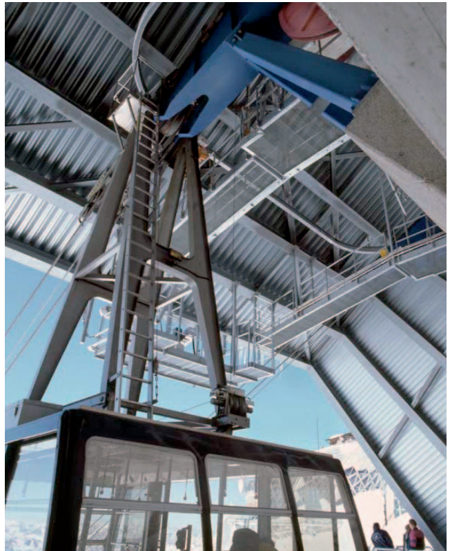
Cable cars: cable sheaves or return pulleys
