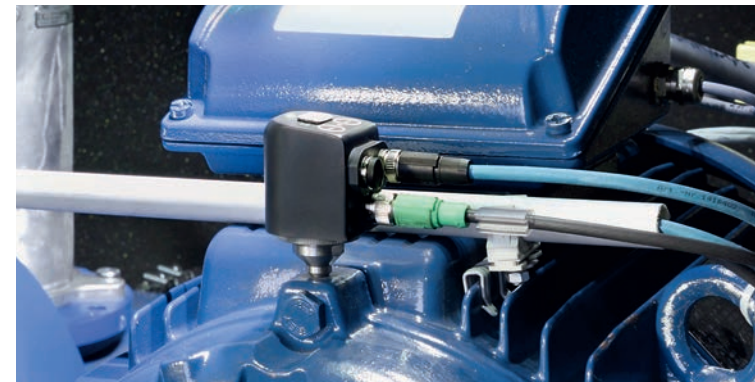
Reduces unplanned downtimes: Online condition monitoring with FAG SmartCheck
