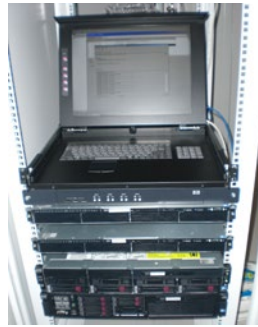
Server arrangement on site
