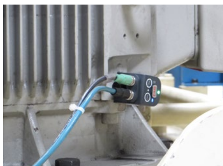
FAG SmartCheck at the base of one of the drive motors
