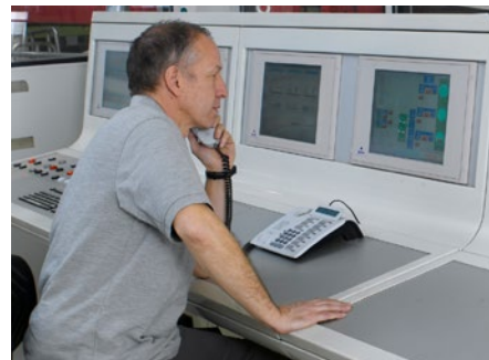
The customer-specific visualization allows the operator to monitor the system easily
