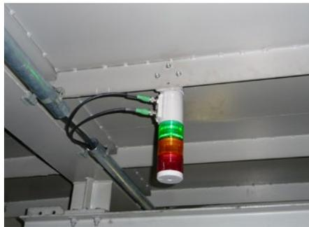
Simple visualization of the operating condition with the help of the FAG SmartLamp
