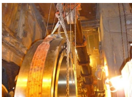
Fitting of non-drive spherical roller bearing
