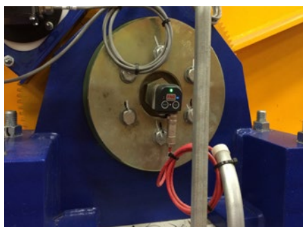
Monitoring of drive elements using the FAG SmartCheck
