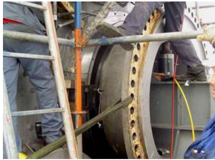
To remove the inner ring segments of the old bearing special tools were made
