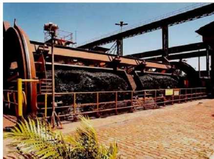
Pelletizing plant to fill the preformed pellets into the pellet cars
